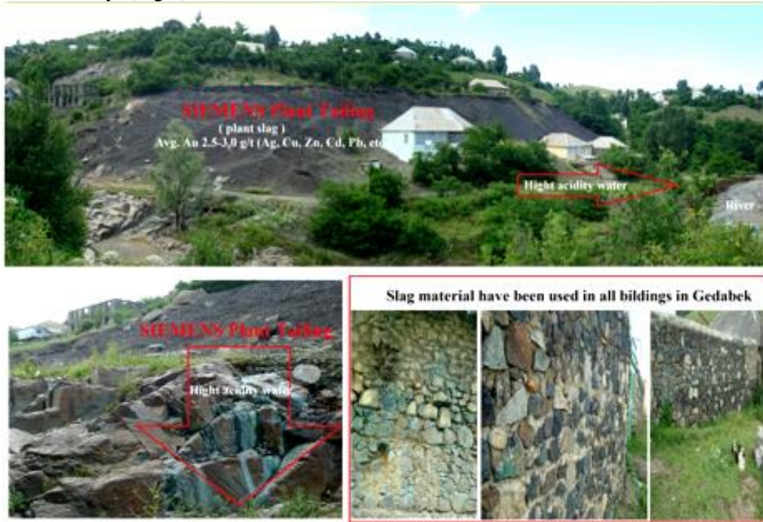
Fig. 7. Gedabek city. Locals houses built on the tailings area. Slag materials applied at the houses construction.
