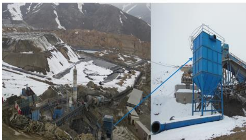
Fig. 3. Old crusher and dust collector.
